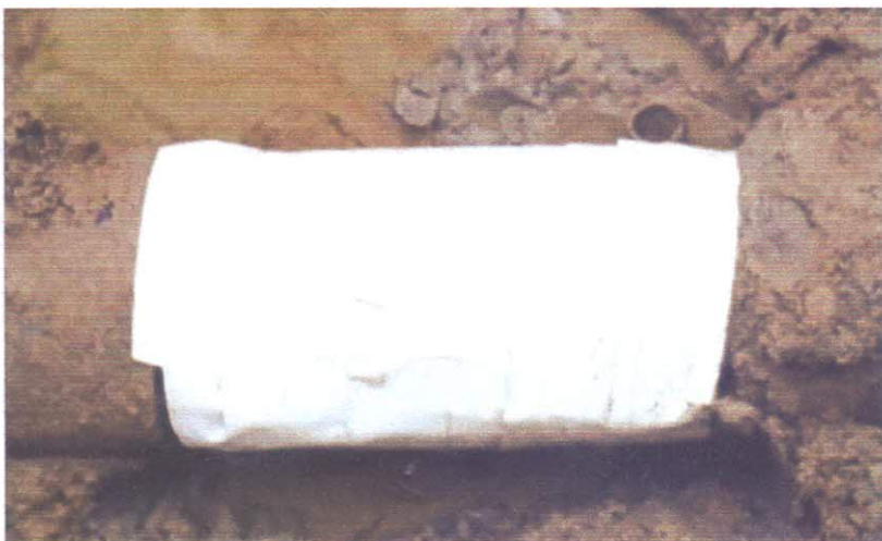
Picture of the Point B on the Facility (After repair)
