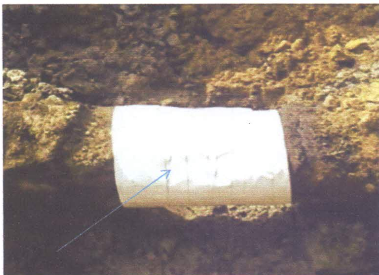
Hacksaw cut on the Facility at Point A (After repair)
